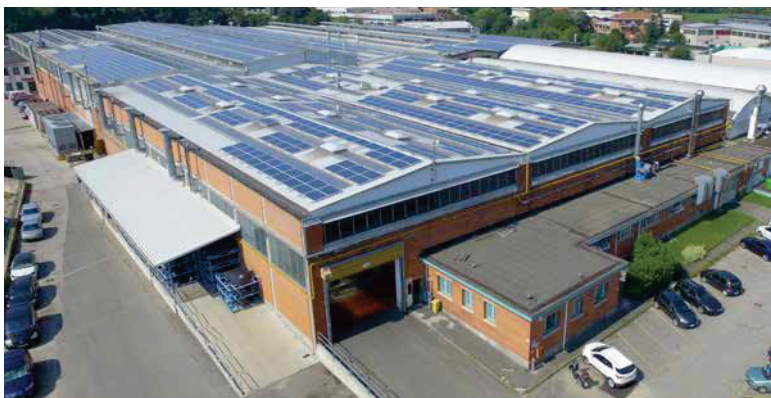
Cornaglia Facility - Photovoltaic systems
